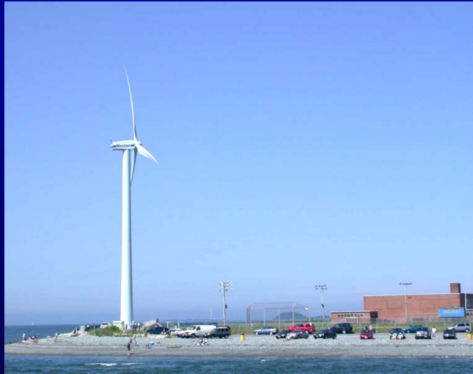
Hull's 660 kW turbine next to high school (Hull, MA)
