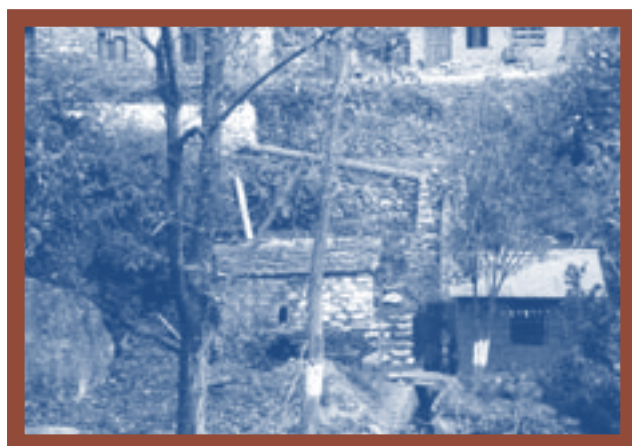
Improved Micro-Hydro site for electricity generation, India. (© IT Power)
