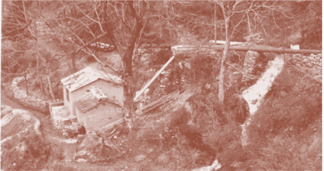
Improved Micro-Hydro site for electricity generation, India. (© IT Power)
