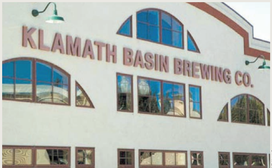
The Creamery Brewpub and Grill is one of the case histories described in UGWG workshops. It uses geothermal energy from the Klamath Falls, Oregon, geothermal district heating system for all its heating purposes. Uses of geothermal energy include space heating of approximately 11,000 ft 2 (1,022 m 2 ) of restaurant/pub space, snow-melting of about 1,000 ft 2 (93 m 2 ) of sidewalks, and generation of hot water for the brewing process. In cold months the brewery saves about $1,100 in space heating expenses and saves around $300 per month in energy used to brew the beer.
