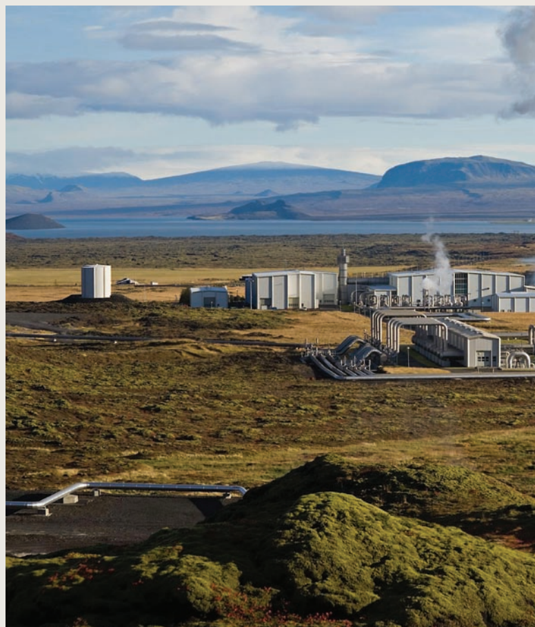
The 120 megawatt Nesjavellir Geothermal Power Plant in Iceland.
