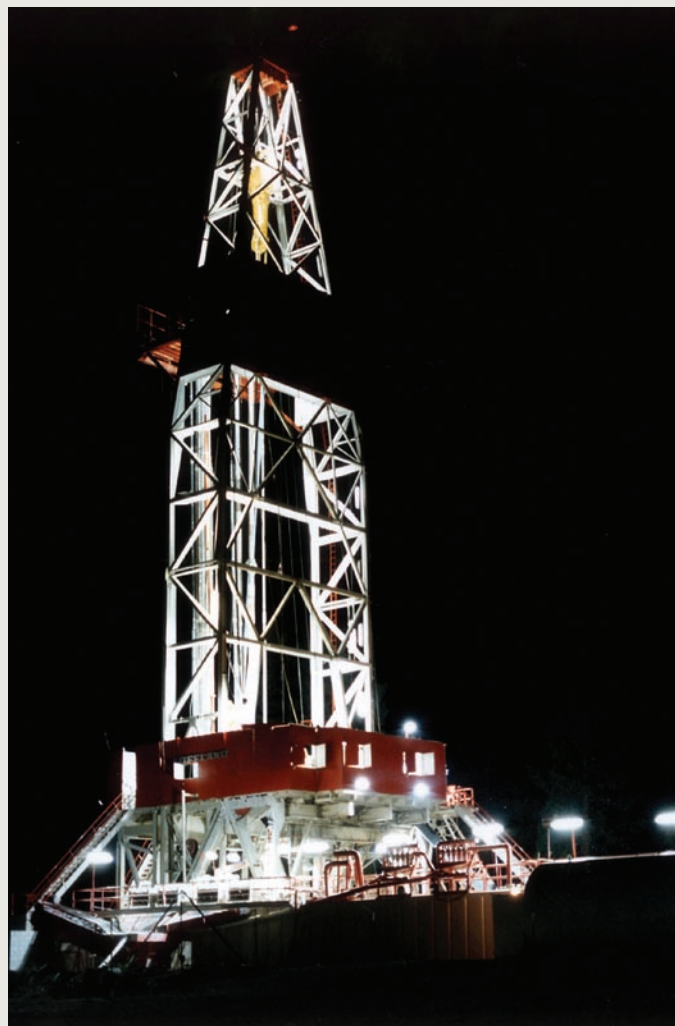
Geothermal well drilling at the Long Valley Exploratory Well near Mammoth Lakes, California.
