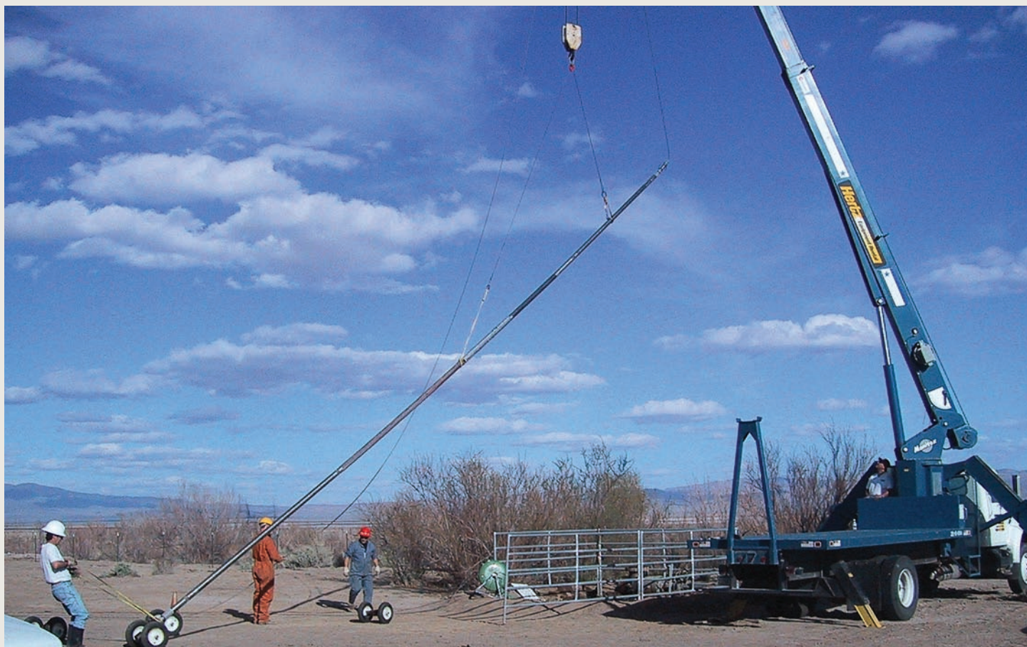
GeoBILT EM Induction logging tool being deployed at Dixie Valley.
