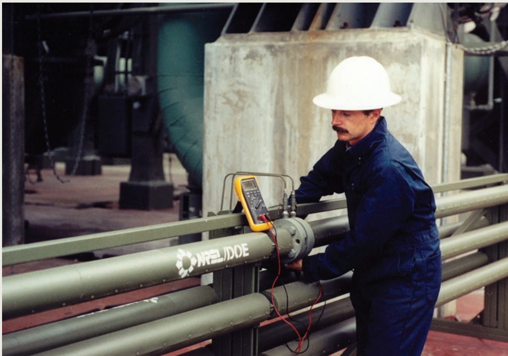
Keith Gawlick, of the National Renewable Energy Laboratory, field testing coatings at the Mammoth Pacific Geothermal Power Plant in the Sierra Nevada Mountains.
